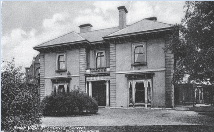
Coventry Hall, Streatham as St. Andrew's Convent in the 1970s, before eventual demolition
